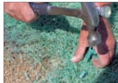
Install using DeWitt biodegradable E-Staples
