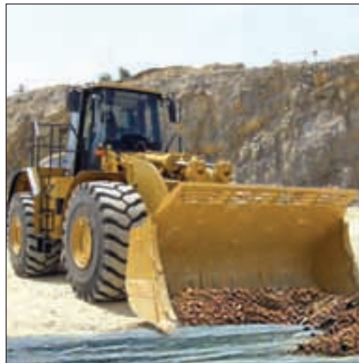
Woven geotextile installation
