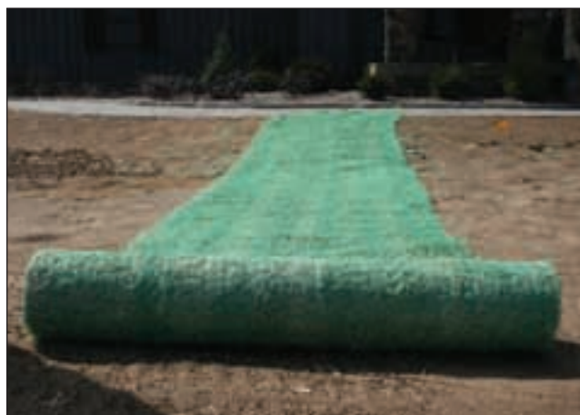
Erosion blankets are easy to unroll and install.
